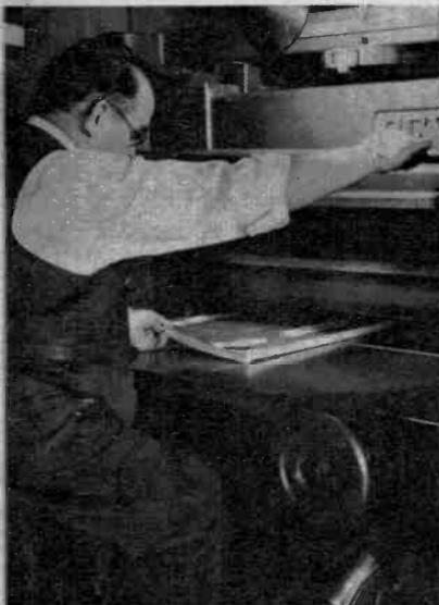
**9** Card designs are printed on sheets measuring 3x4 feet, then cut smaller by Walter L. Dickinson (above)
