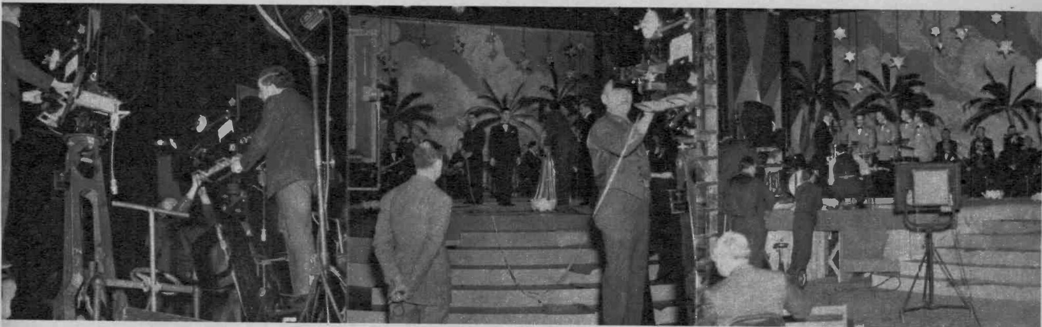
Two cameras, on movable trucks for better shooting-angles, are used in filming a picture, the best print of the scene being used when the picture is assembled
