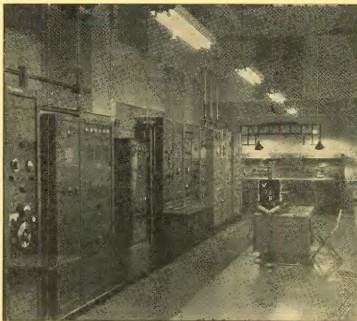
THE 10,000-WATT transmitter of W7INY, owned by station WOR, is located on the top floor of a skyscraper in midtown New York City. W7INY, the second FM outlet in the nation to begin commercial operation over a year ago, serves an assigned area of 8,500 square miles
