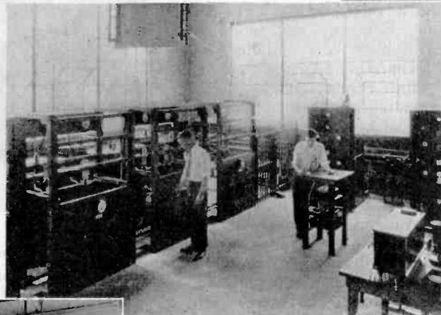
At the left are shown three modulator units, each with a group of water-cooled tubes, and audio frequency amplifier units at WGY
