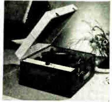
A new portable automatic record player in a two-toned leatherette carrying case. Holds the single post VM Record Changer; case also includes three tube moist amplifier and P. M. speaker.
