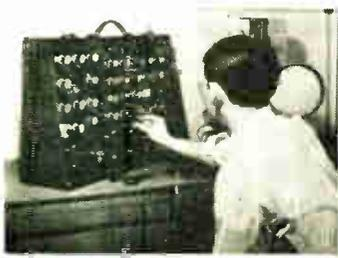
The composite video generator brings to the service engineer in a single, small portable case all the elements needed to provide a complete "standard television video signal." This makes it possible for trouble shooting or repair work to be carried out in the shop or in the home, at any time—and no time is lost waiting for a television transmitter to come on the air.
