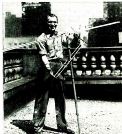
A few seconds later and Dick snaps the high frequency dipole into position. It costs only 6¢ in labor to assemble this Ward Minute Man antenna.
