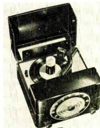
In a plastic cabinet less than a foot square, this radio-phonograph combination has a two-speed motor, operating automatically at 33-1/3 and 45 rpms. Has single tone arm and two center posts, each holding up to 10 records. Radio is a 5-tube super-heterodyne circuit, with beam output, automatic volume control and built-in antenna.
