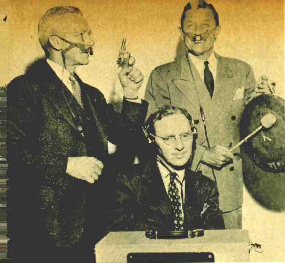
▲ **THE ARMY'S "LIP MICROPHONE"** is here being demonstrated by Parks Johnson (left) and Warren Hull (right) on CBS' "Vox Pop" show, to prove that such outside noises as pistol shots and gong-ringing need not interfere with transmission of human voices over the radio. At the controls of the battle-tested device is R. G. Thompson, Columbia's Eastern Division Operations Engineer.
