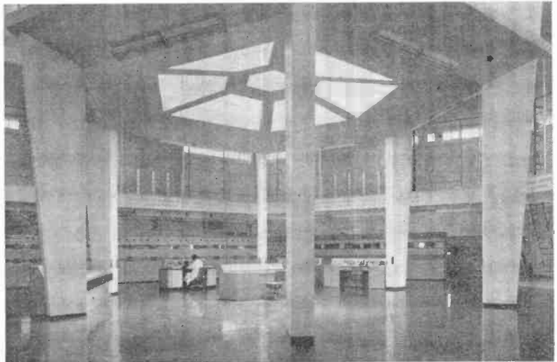
This is the impressive transmitter building of "Radio Vaticano," Vatican City.
