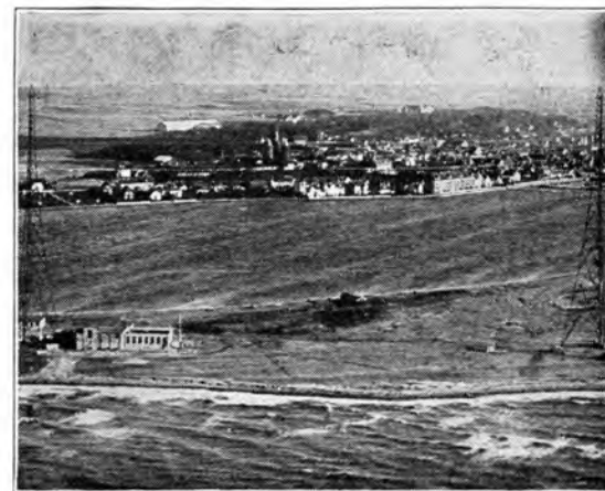
AERIAL VIEW OF KALUNDBORG STATION
