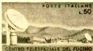
Italy 1968 Fucino Installation
