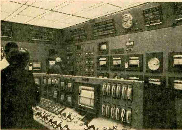
Above, output transformer at San Onofre; below, master control room. Indicator panels continuously flash status of instruments and equipment to engineer in charge; levers control position of rods in core.
