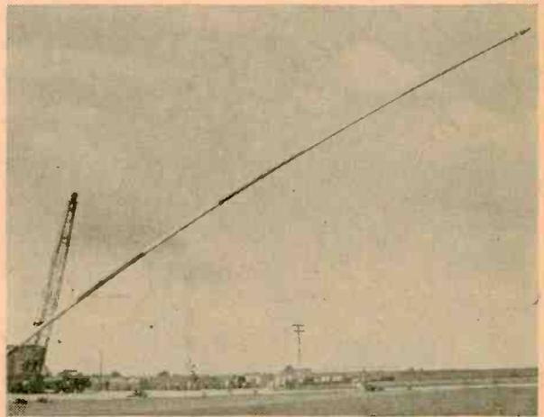
Breathtaking part of 20-minute erection time came as 225-ft pole was progressively raised higher and higher toward true vertical. As safety precaution, steel cable was placed around pole near base and held taut by winch truck. Erection crew found plenty of opportunity to put their two-way radios to good use during course of actually raising 26,850-lb. tower.
