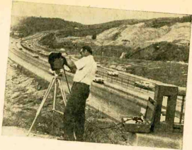
... clouds of nitrogen dioxide were recently studied remotely by a team of Canadian scientists? Working under an HEW contract and using a unique, telescopic, gas-analyzing spectrometer, Toronto's Barringer Research Inc. was able to perform quantitative chemical analyses of polluted air over the Los Angeles basin without making physical contact with the material under study.
