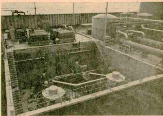
Steam generators and turbine generator (left) form secondary portion of generating setup. Though heated by nuclear energy, pressurized water serves only as means of conducting energy between reactor and steam generators. Right, sea intake and outflow pump pit.
