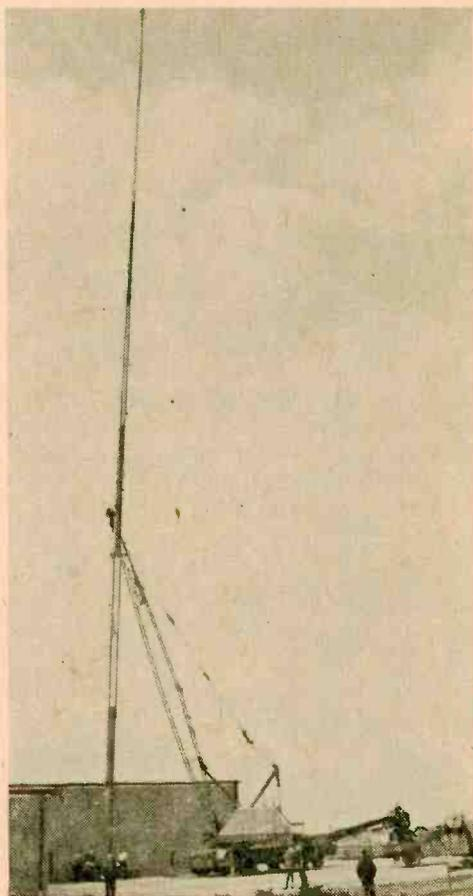
Coop engineer Wiley Jones (sweater) checks pole position over anchor bolts before pole is lowered into final position. Once pole had been seated on anchor bolts, workmen then adjusted first leveling nuts, then anchor nuts to ensure that entire 247-ft-high structure was both adequately secure and accurately locked in true 90-degree-from-horizontal position.
