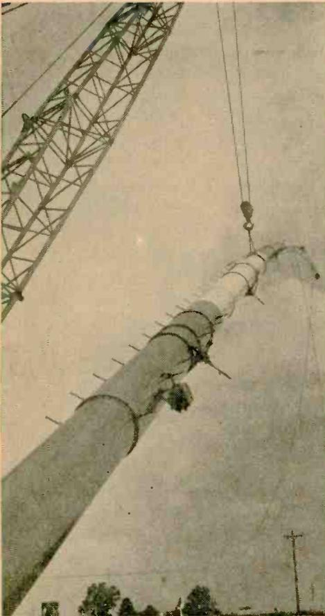
pole was assembled and painted, and the aircraft warning lights installed and wired. The three lower sections had the wire rope slings in place with the come-a-longs (coffin hoists) in tension. Before raising the pole into position, a tag line was fastened at the top of the pole and another one about halfway down. Taking care to protect the aircraft warning light at the top of the pole, workers fastened the wire sling at the balance point of the pole.
