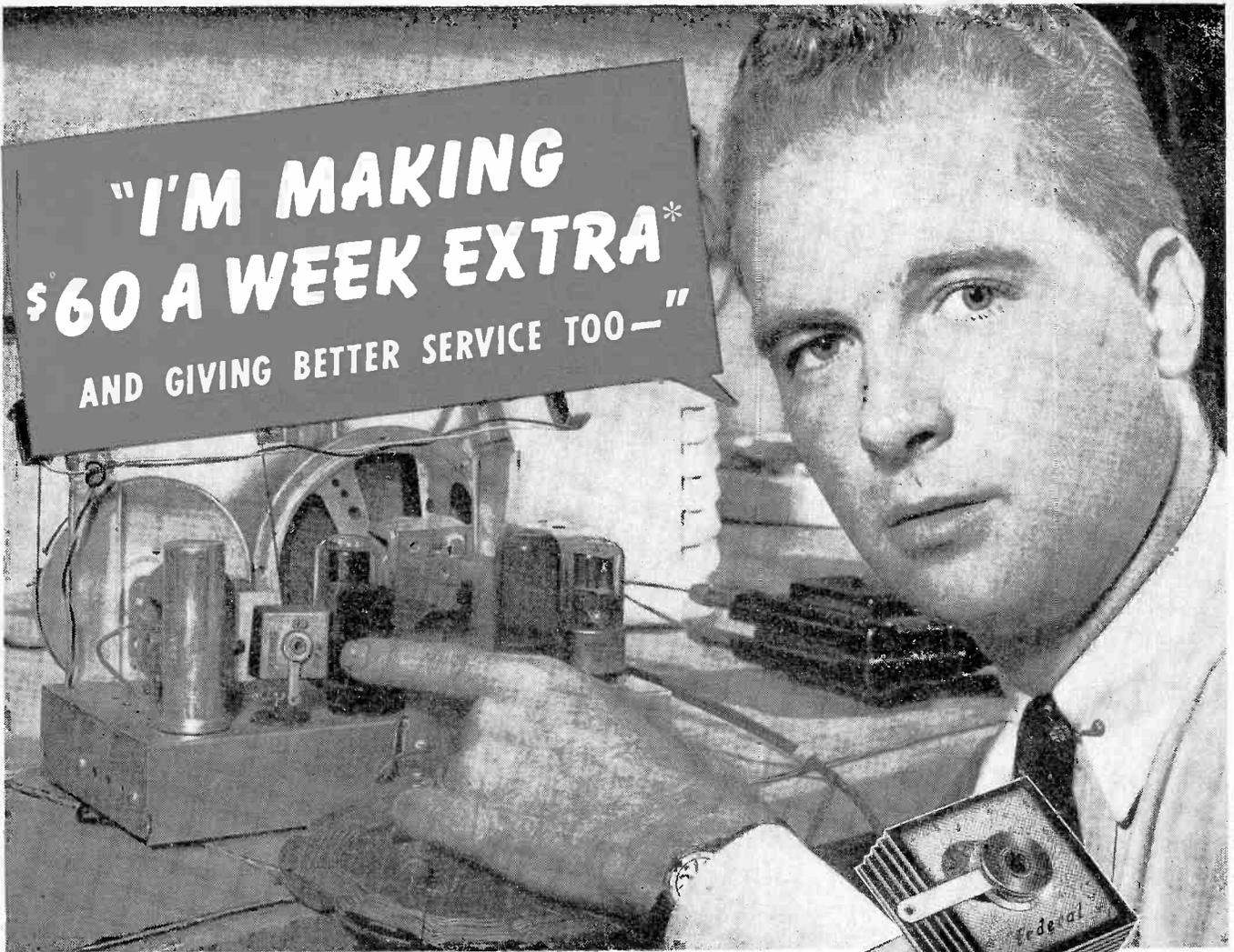
**by Installing Federal's Miniature Selenium Rectifier—in AC-DC home radio receivers to replace rectifier tubes**
