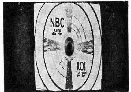
Fig. 8 A test pattern showing the effects of an incorrectly set horizontal width control.
