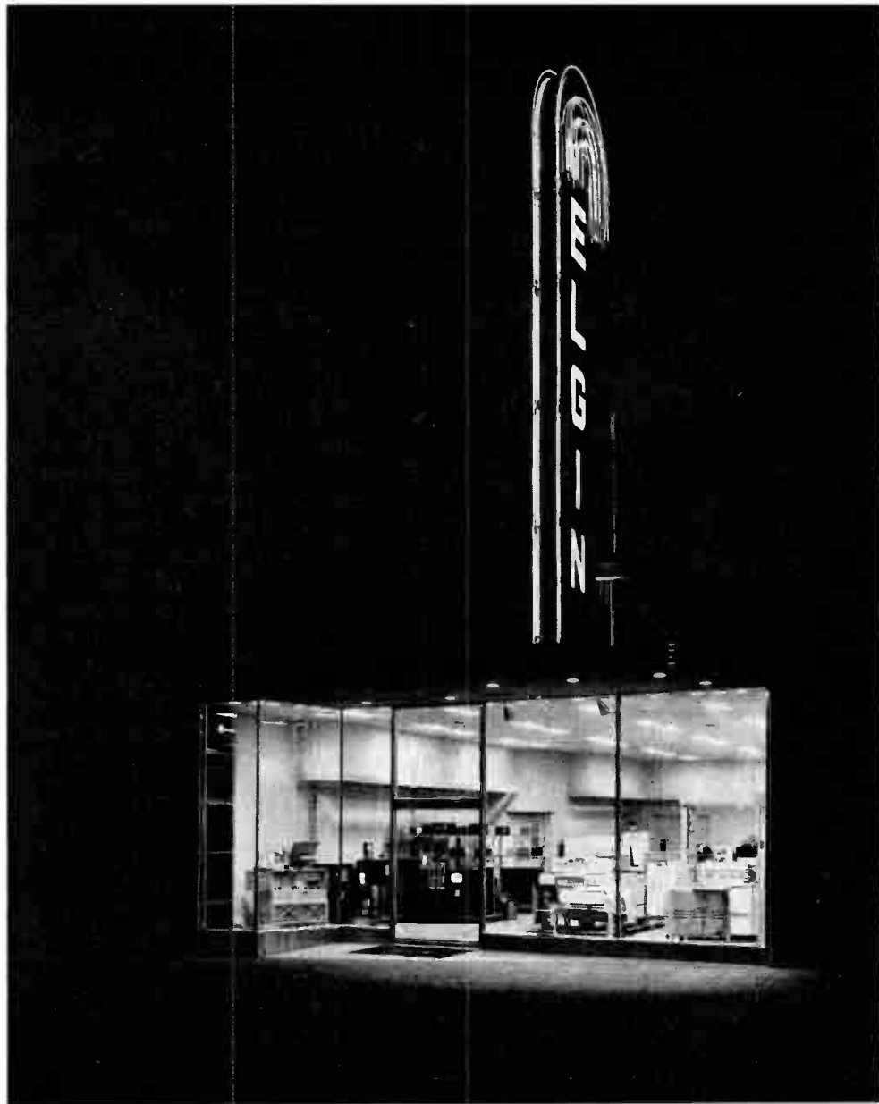
An excellent example of the use of glass and light for an attractive store front. Notice how modern effect is achieved. (Photograph courtesy Pittsburgh Plate Glass Co.)
