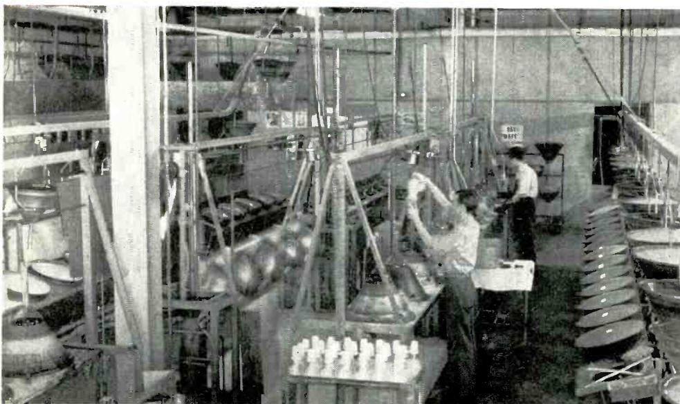
Depositing screen material on face of tubes. After screen has been deposited, solution is decanted. The tubes just left of center, appearing somewhat blurred, are in the process of being decanted. Both natural glass and dark faced tubes are produced, although DuMont receivers do not use the dark-faced variety.
