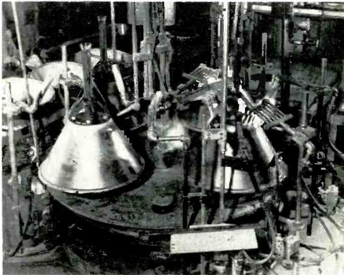
In the pictures that follow, the essential steps in the production of picture tubes are illustrated. At left, one of the first operations is executed: sealing metal cone to glass neck. These tubes are of the short-neck, metal variety. Dr. DuMont foresees larger direct view tubes. He considers a 4 x 5 ft tube very likely.
