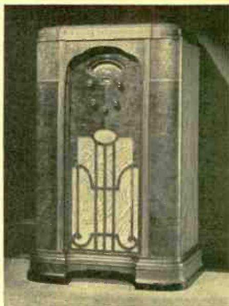
**ALL WAVE**—Model 112N—Scientific high fidelity tests show that this is the finest radio that we ever built. Other sets cost much more, but we know of none that matches the performance of this 12-tube All-wave Kent. 10-kilocycle selectivity over entire tuning range—15 watts undistorted output—4 tuning bands—540 kilocycles to 18 megacycles—bass compensation—true high fidelity reproduction. **\$165.00 f.o.b. factory.**
