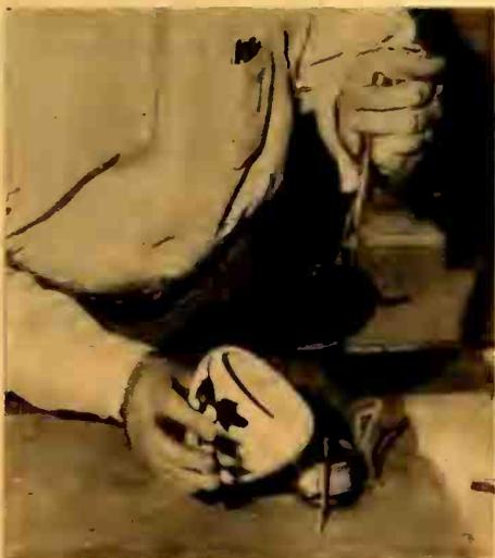
**3. The hot, blackened paraffin is carefully poured to cover the entire bottom and seal up the crack.**
