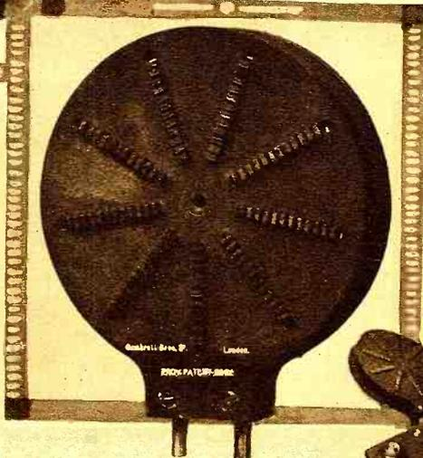
Left: A fixed inductance coil of the multi-layer type with plug attachment. An air space is left between each layer similar to the Morecroft inductance. Below: A small receiving set employing three of these coils.
