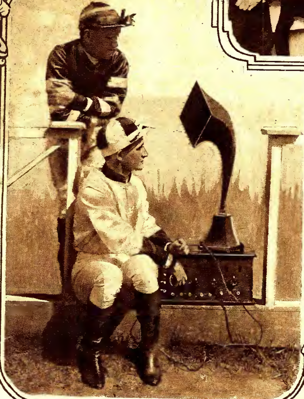
Left: Jockey Burns tunes in for Thurber just before the races at Belmont Park. The set employs two stages of radio frequency amplification, a detector and two stages of audio frequency amplification. © Foto Topics, Inc.
