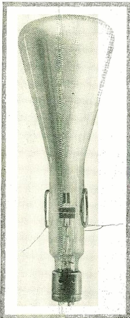
A commercial form of cathode oscillograph with coils attached for obtaining characteristic curves of vacuum tubes.
