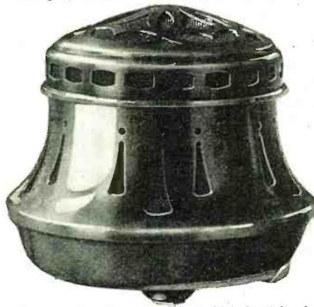
A German loud speaker, for which is claimed remarkable reproduction, is shown above. It is built on reflected tone principle.
