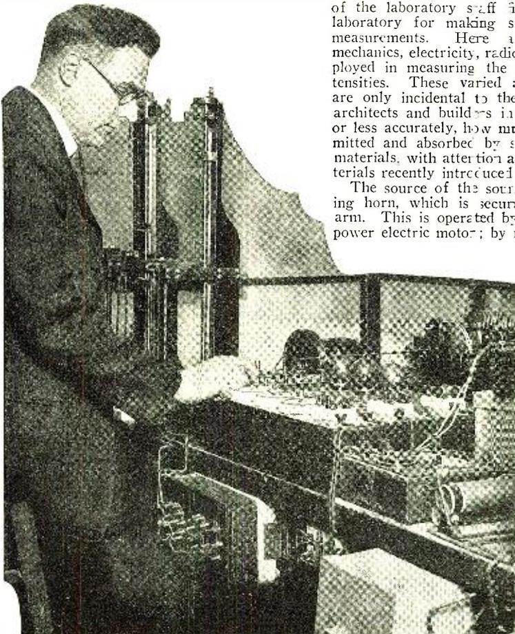
The three tubes of the three-stage audio frequency amplifier may be seen in the photograph at the left. After passing through the amplifier the signals are rectified by a crystal detector and comparative readings are taken on the galvanometer.
