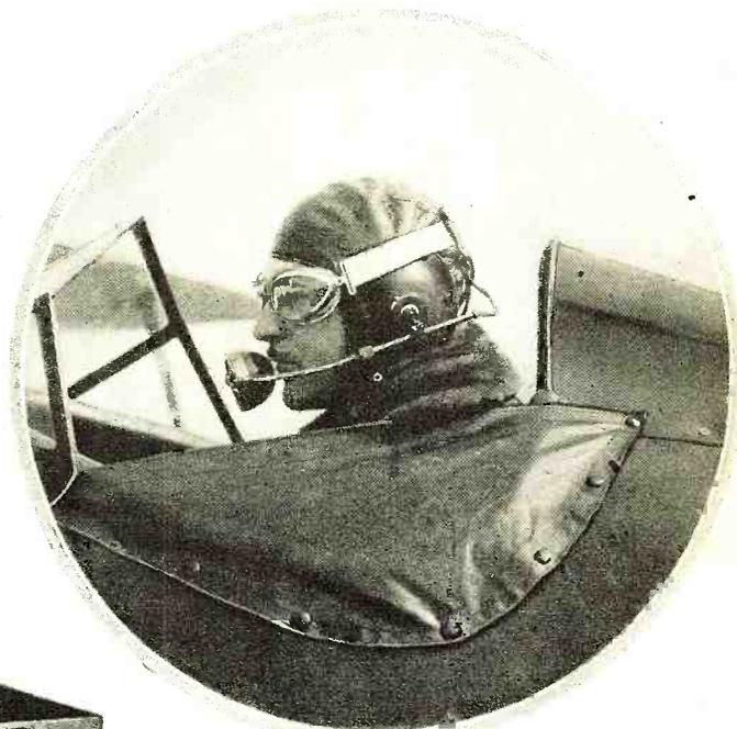
The microphone used by mail pilots is attached to their helmets in the manner shown above. Operation of the plane-to-ground communication system is easily conducted—the pilot merely changing from transmission to reception by turning the switch
