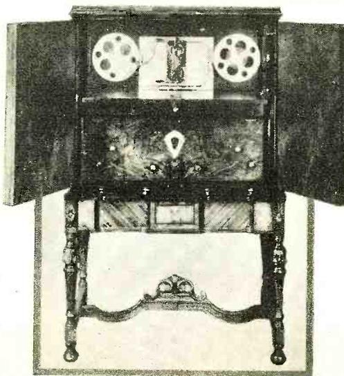
The Victor Animatograph 16 mm. projector and turntable, at the lower left—a unique arrangement where the turntable is geared to the horizontal shaft of the projector and the turntable assumes a vertical position instead of horizontal. By means of a sliding counterbalance the weight of the individual pick-up head used can be neutralized. A spring keeps the pick-up pressed against the groove in the record
