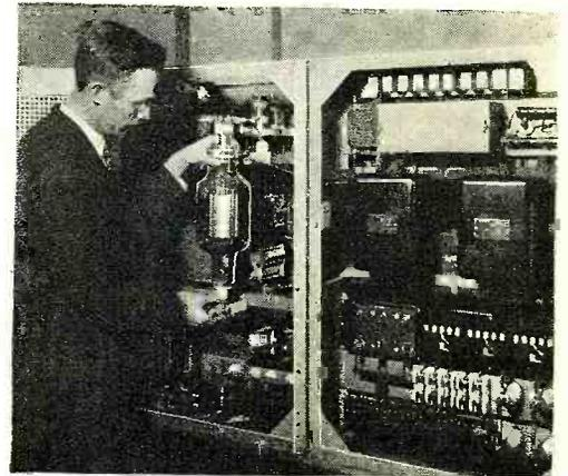
Shown above is the rear of the rectifier and oscillator panels of the transmitting equipment installed in the ground station
