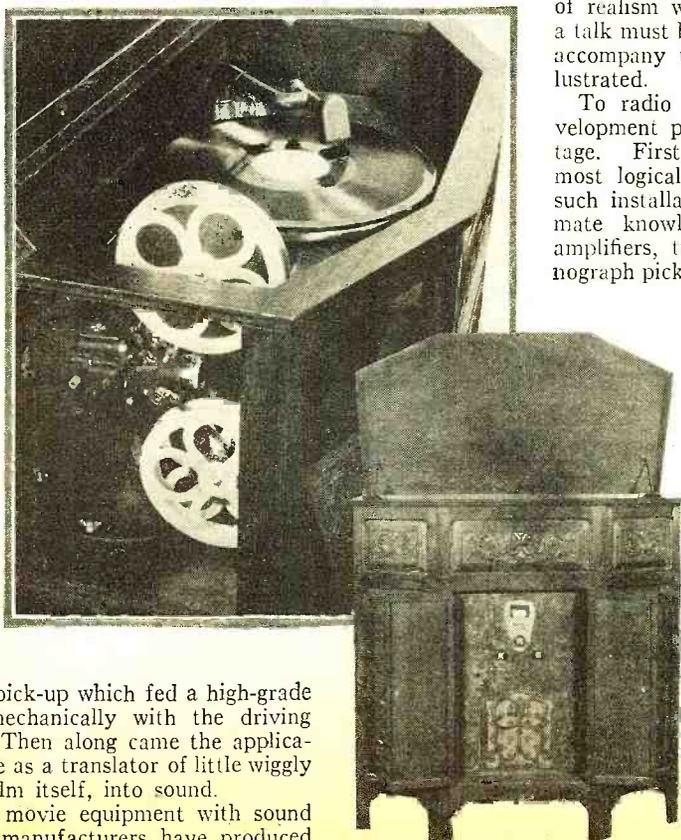
The Bell and Howell Filmotone, a combination radio and home talking movie outfit. The lower illustration shows the general appearance of the pretentious cabinet, with radio receiver in the center portion, while the upper illustration shows the arrangements of the turntable and the projector
