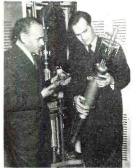
Two high power television tubes. The plates become so hot that water cooling is needed.
