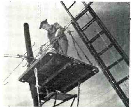
Outdoor experience in cable repair and service at the Training Center.
