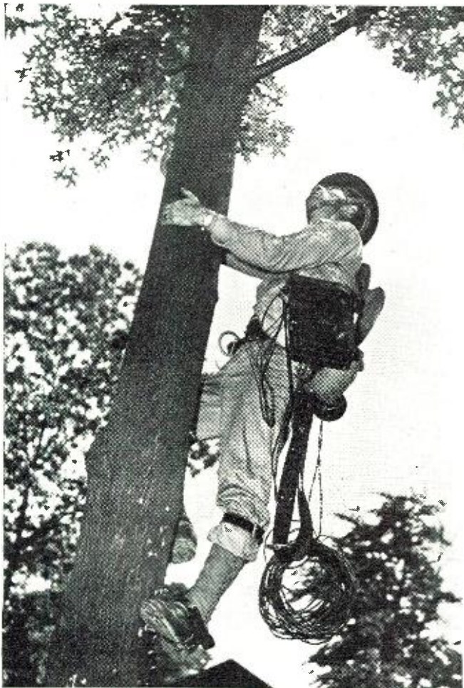
This lineman is ascending tree where he will make an overhead wire crossing. This job requires great skill.
