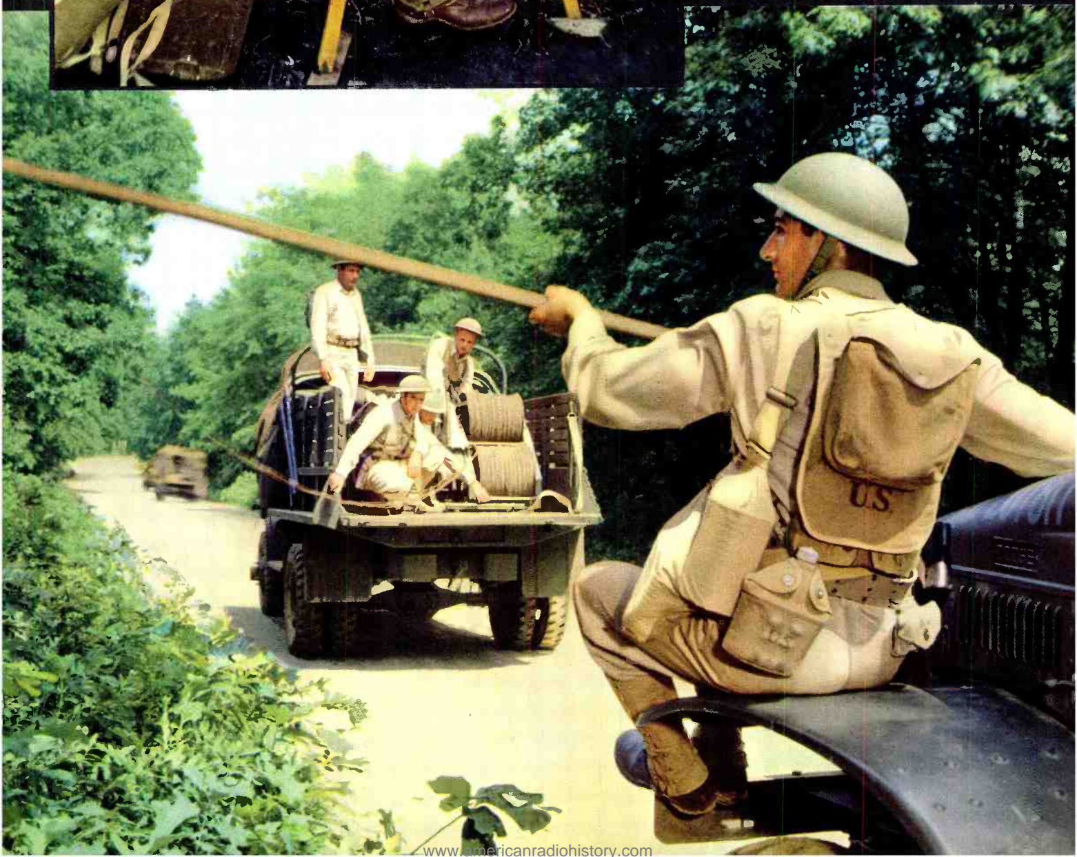
Guiding telephone wire away from road. Truck ahead feeds thousands of feet in one hour.
