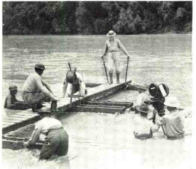
Signal Corps Training Film Field Unit No. 1, photographing details of foot bridge construction, Ft. Benning, Georgia.
