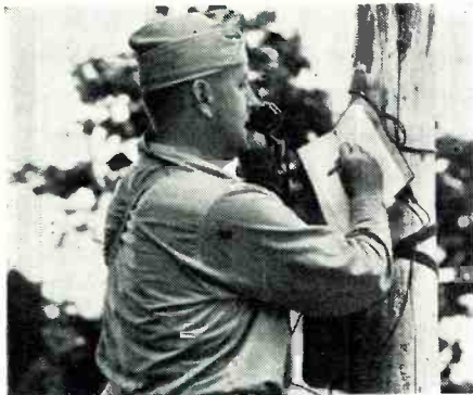
Outpost field telephone straps around pole or other supports.
