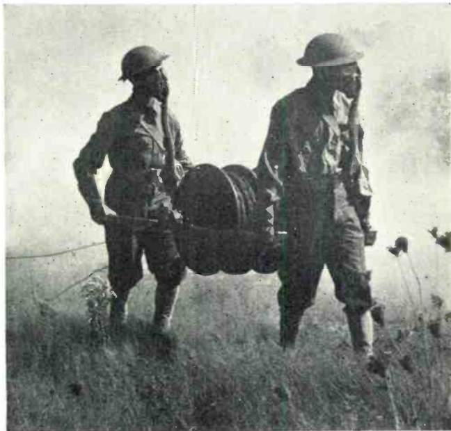
Communications are vital to the success of any operation. Even gas attack cannot halt the process of laying cables.
