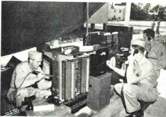
This group of different types of portable and field switchboards undergoes inspection by students.
