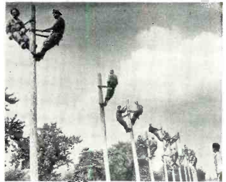
Instruction in pole line construction at Signal Corps Schools.
