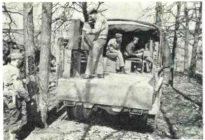
Complete telephone switchboard and signal center. Temporary terminal board is connected enroute.
