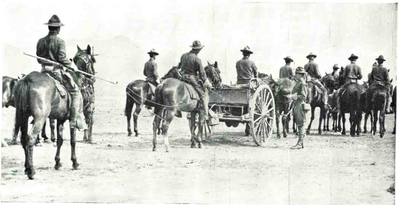
Playing out field wire from horse-drawn wirecart, 1913. Soldiers of the Cavalry rode behind to guide wire as it was fed from the preceding cart.
