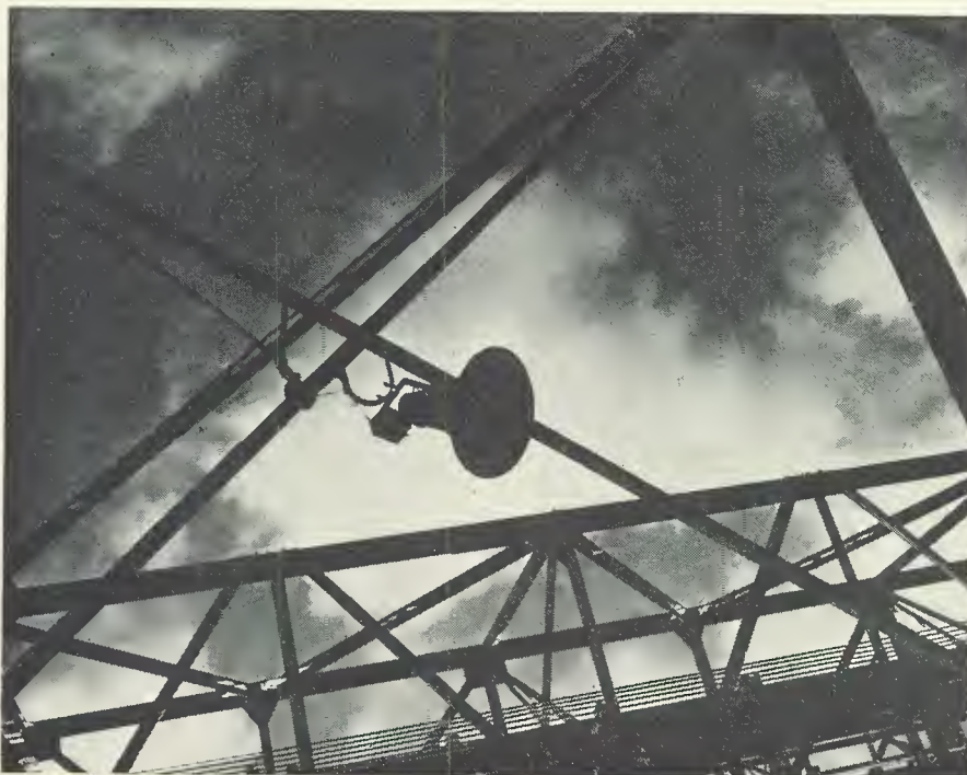
This speaker is installed in the steel framework on ways for new battleship U.S.S. Alabama.
