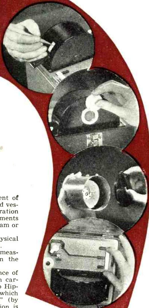
Fig. 1. The Stetho-Cardiette instrument produced by the Sanborn Company. It provides simultaneous or separate stethogram and electrocardiogram, plus amplified auscultation. The circular inserts show various views of the photographic film chamber.
