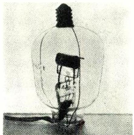
were used in this amplifier, the second being a de Forest Audion. The amplifier, which is shown in Fig. 213, was of the high frequency type using regeneration, and was intended for use in connection with the Mark III Short Wave Tuner.
