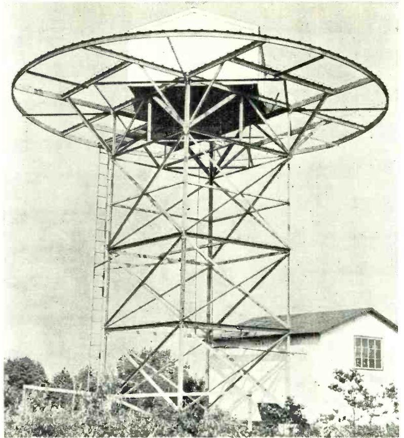
Antenna house and tower. Within the house are located five antenna loops. A wide apron effect is produced by steel wire mesh counterpoise.
