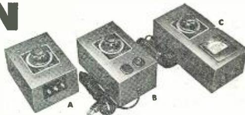
The UTC Varitran is a simple autotransformer whose turns are arranged on one layer with the insulation removed so that every exposed turn may be used as a tap of the winding. A special non-fusing contact, having resistance to minimize circulating currents, is mechanically arranged so that it can be moved to any position on the winding, permitting the exact voltage desired to be obtained.
