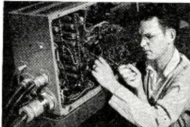
Rear end of RCA modern television monitor and control unit. Four types of Cannon Plugs are used in this unit: "TQ", "P", "K" and "FMRP".
