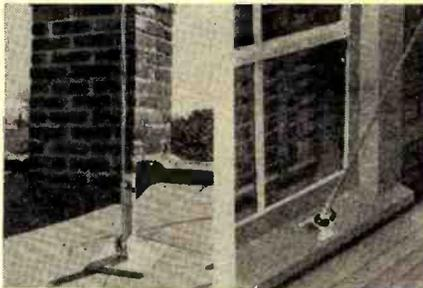
various roof positions including installation on the soil pipe. The mast may be collapsed to four feet for easy handling.
