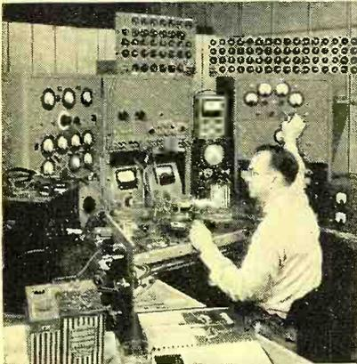
COVER PHOTO: Don Zunker, Central lab engineer, checks a new amplifier unit which incorporates the company's Printed Electronic Circuits in the development and test laboratories of Central Lab, Division of Globe-Union in Milwaukee. (Photo by Moni Hans Zielke)
