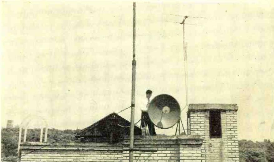
Engineer Tom Humphrey makes an adjustment on the studio-transmitter radio link microwave dish antenna which beams programs from atop the Ithaca Savings Bank Bldg. to Connecticut Hill, whence they are channeled to six other stations in net.
