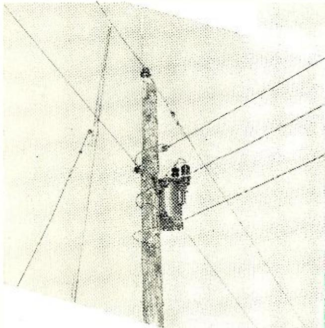
Fig. 1. Two views showing "hot stick" method of coupling mobile unit to the power line for carrier communication transmission.
