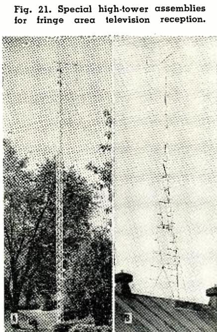
Fig. 21. Special high-tower assemblies for fringe area television reception.
