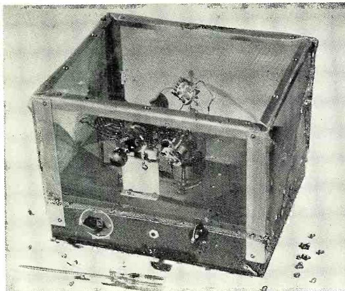
A solid bottom pan can be used in place of the wire screen.
