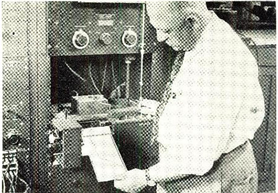
Fig. 4. Automatic recording of frequency response curve of speaker of Fig. 1.
