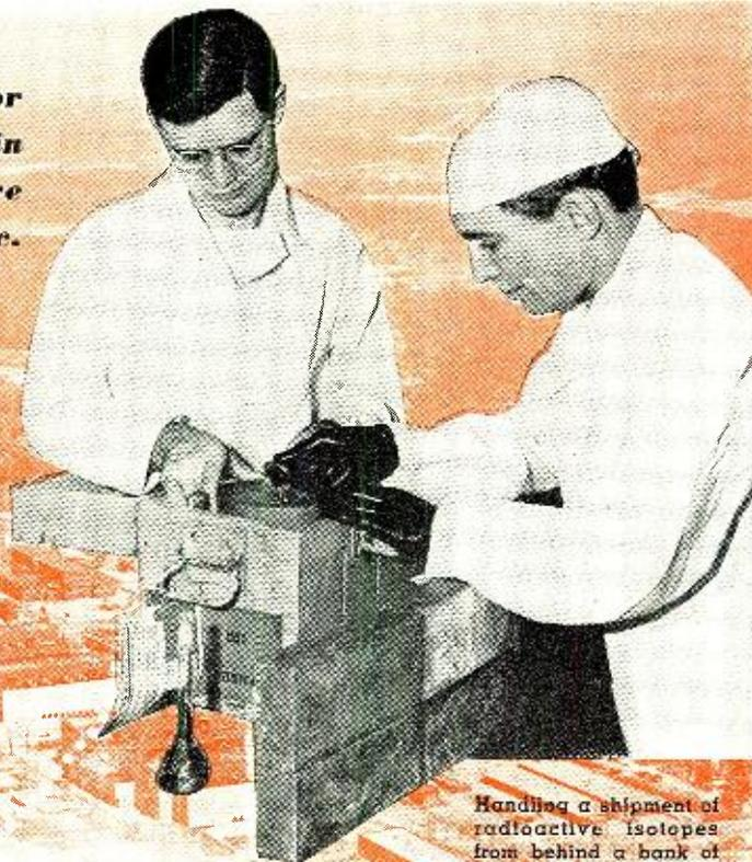
Handling a shipment of radioactive isotopes from behind a bank of lead bricks as a safeguard against exposure to radioactivity. Background shows bird's eye view of Y12 electromagnetic plant at Oak Ridge, Tennessee.
