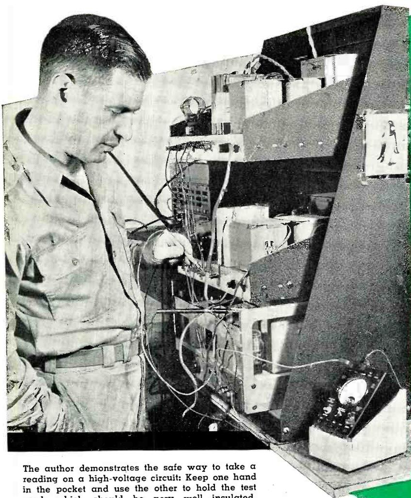
The author demonstrates the safe way to take a reading on a high-voltage circuit: Keep one hand in the pocket and use the other to hold the test prod, which should be very well insulated.
