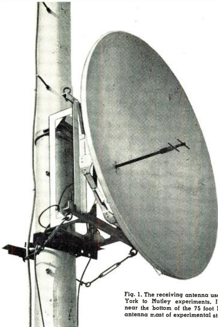
Fig. 1. The receiving antenna used in the New York to Nutley experiments. It is mounted near the bottom of the 75 foot FM broadcast antenna mast of experimental station W2XFZ.
