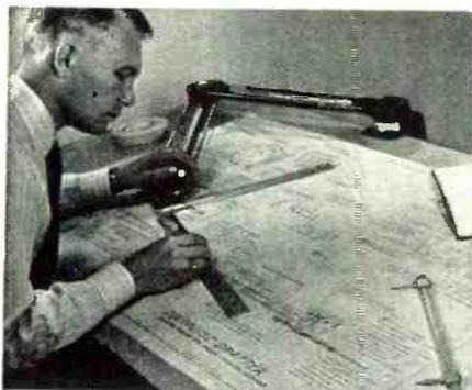
tion and hold it. Other features are a base line clamp for greater convenience in aligning the drafter to the drawing, ball joints on both arms for flexibility, and increased space between the double thumb screws that improve anchorage.
