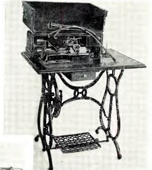
Fig. 8. The improved Edison "treadle phonograph" for office dictating.
