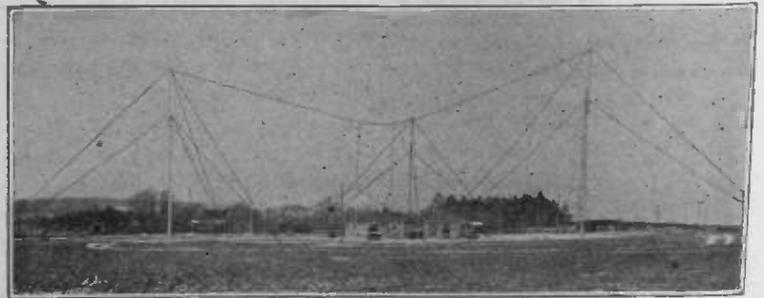
Fig. 4. Wooden Masts Must be Used for the High Speed Waves, as Shown Here
