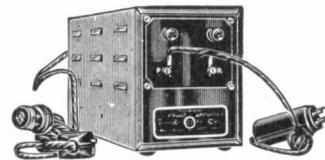
a complete "B" Eliminator furnishing all the "B" current required by the regular tubes of the set. No adjustments required and no output transformer or similar auxiliary equipment needed with either unit.
