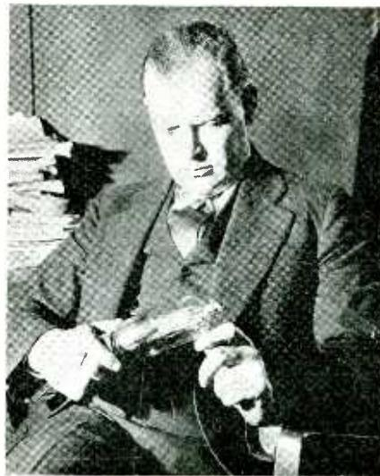
The "birdie" at which Allen B. DuMont is staring so intently is an electron motor vacuum tube, pride and joy of DeForest's chief engineer. The grid can be made to rotate, suggesting a number of commercial possibilities, by applying proper filament, plate and grid potentials.
