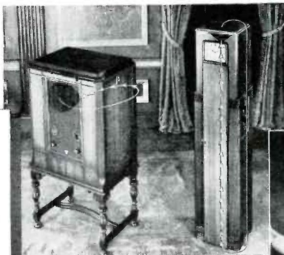
HERE'S THE LONG BAFFLE. The shorter the baffle, the fewer low tones you hear. Notice the difference in baffle in standard style cabinets (left) and the "Columaire" (right).
