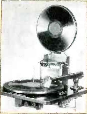
Model 10-12 in loading position. Note the lever on right side which throws the unit into position for 10-inch records when down or 12-inch records when up. With a special arrangement incorporating a double-throw master switch, one record can be placed on the turn-table, the adjustment set according to the size of the record and the magazine can be loaded while the pick-up automatically comes into position and the first record is being played.
