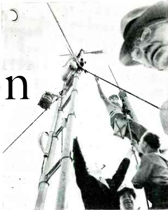
● *Completing the television antenna and lightning arrester on top of the airship mooring mast, 1,250 ft. above the sidewalk*
