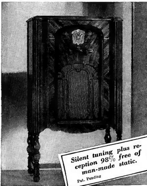
Model K-120 - Completely shielded 8-tube console superheterodyne. Automatic volume control. Latest type radiotrons; R. F. and A. F. Pentodes. Phonograph pickup connection. Outlet for Kolster 3-tube short wave converter. Full 8 1/2-inch dynamic speaker. Cabinet, 41 inches high, carries cross fire butt walnut panel, zebra wood top and bottom rails and pilasters. Price (with Radiotrons), \$74.75.
