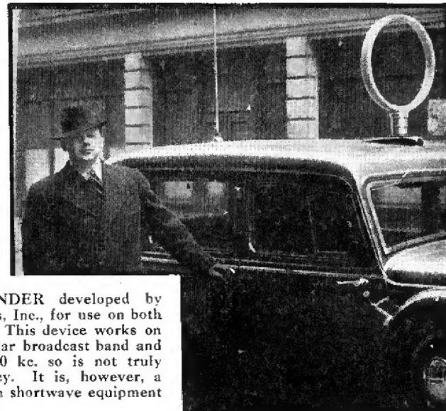
DIRECTION FINDER developed by Lear Developments, Inc., for use on both aircraft and ships. This device works on signals in the regular broadcast band and from 3,000 to 6,200 kc. so is not truly ultra-high frequency. It is, however, a new development in shortwave equipment
