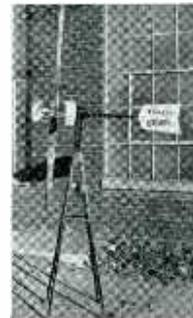
wood construction—wood to keep it light in weight and edges reinforced with metal strips to resist rain, sleet, sand or any flying objects in the wind. It is controlled with a flap-type governor which is operated by propeller speed rather than by wind pressure.
