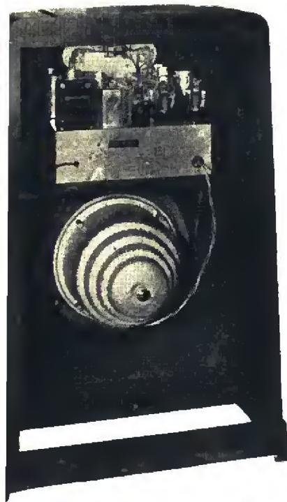
**INDIVIDUALITY . . .** Over the back of the speaker in this receiver is a cover comprising two concentric sections, plainly visible to the consumer. Low frequency response may be adjusted to fit rooms by varying the rings
