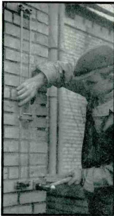
▲ SPEED . . . Adjustable prick-punches built right into a jig save much time when positioning holes to hold mounting flanges and straps for iron-pipe masts
