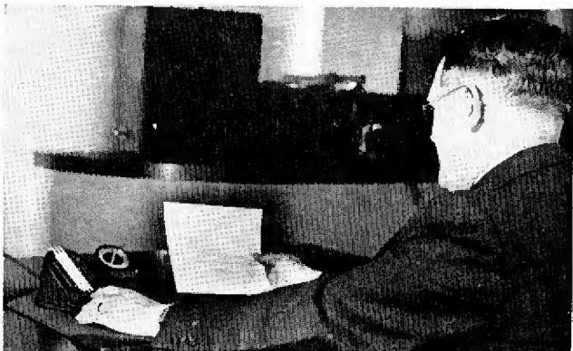
COMPACT CONTROL—This new and novel unit with a 45-degree angle case comprises speaker, mike and switch. An external amplifier is used. (Sound Systems, Inc., Cleveland)
