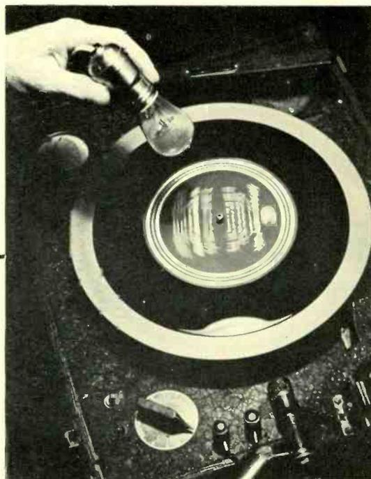
**CHECK TURNTABLE SPEED**—True tone cannot be obtained unless recording and playback are exactly synchronized. Simplest accurate check is by means of stroboscope disc and neon lamp
