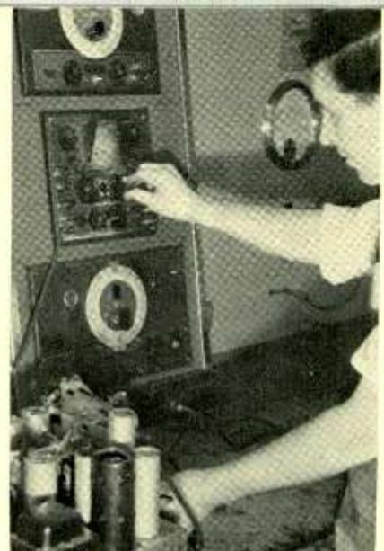
**BRUTE FORCE PLUS BRAINS**—W. C. Siegrist tags intermittents by boosting line voltage with an auto-transformer, watching for part failures on the screen of his oscillograph
