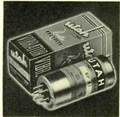
**VIBRATOR**—New line comprising 23 types suitable for auto radio and other services. Latest improvements including vibrator reed with reduced cross section, armature swinging across pole-pieces and double parallel side member frame. *Radio and Television Retailing, June, 1939.*
