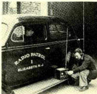
**OSCILLATOR** — Portable oscillator makes it possible to check high frequency signals without removing receiver from radio patrol cars. Can be used for zero-beat frequency check on transmitter. Jack provided on oscillator panel for insertion of earphones. Can generate fundamental signals ranging from 22 to 150 mc. at an accuracy of 1 per cent, is adaptable to use in television, aviation, and other fields employing ultra high frequencies. *Radio and Television Retailing, June, 1939.*
