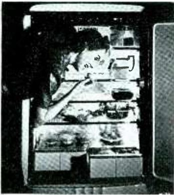
**REFRIGERATOR**—New line of 13 refrigerator models with increased capacity and operating efficiency. Low priced 8 cubic feet model designed particularly for rural use. Deluxe model illustrated shows large shelves and food bins. Equipped with aluminum container for removing food odors. General Electric Co., Bridgeport, Conn.
