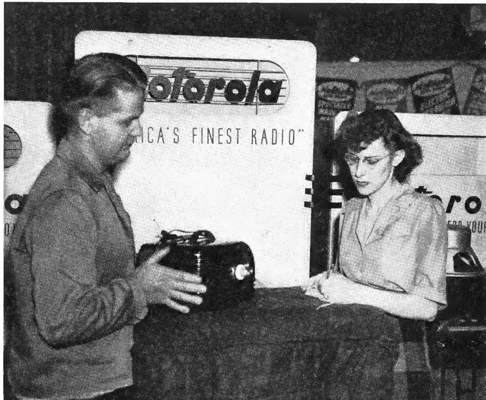
Above, Miss Gould meets a customer and takes the data on the set to be repaired. Below, Mr. De Young checks the set and finds that the trouble is noisy I.F. coils. At right, Miss Gould solders in the new coil and finishes the job by putting the chassis back into the cabinet.
