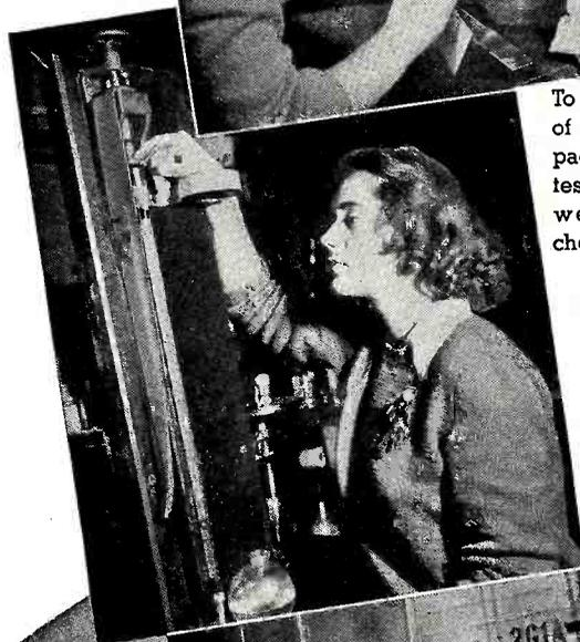
To determine suitability of aluminum foil for capacitor use, every lot is tested for thickness, unit weight and electrochemical characteristics.
