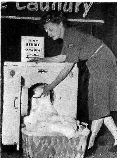
Dryer to be manufactured in electric and gas models. Capacity of 18 pounds wet clothes. Automatic regulator permits removal of clothes dry or damp dry, ready for ironing. Bendix Home Appliances, Inc., 3300 West Semple St., South Bend 24, Ind.—RADIO & Television RETAILING
