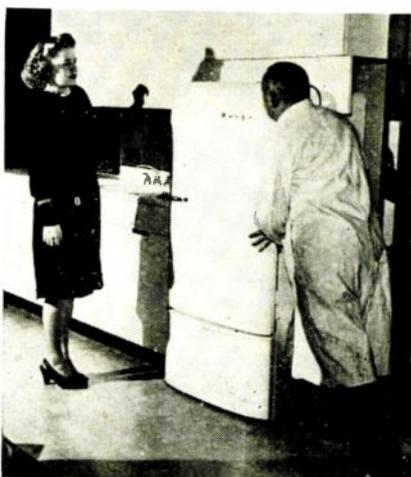
Adaptability of standard household appliances to new prefabricated home utility unit produced by Ingersoll Steel & Disc division of Borg-Warner Corp., is demonstrated by installation of Norge refrigerator in designated space in section.
