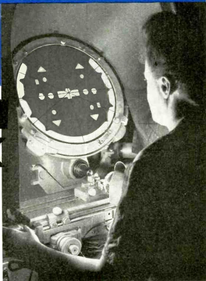
**S**UPPOSE you were given the job of making certain that micas for Hytron tubes were punched exactly to specifications. How would you go about it? You might use a gage or a precise rule. For a modern, faster, more accurate method, however, you would probably choose the illustrated J & L comparator.
